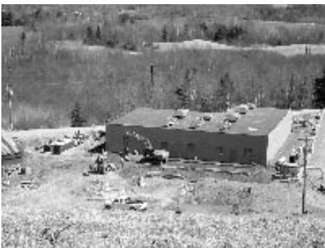
WEC's Landfill Methane Project in Coventry, Vt.
