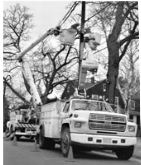
Marblehead line crew at work
